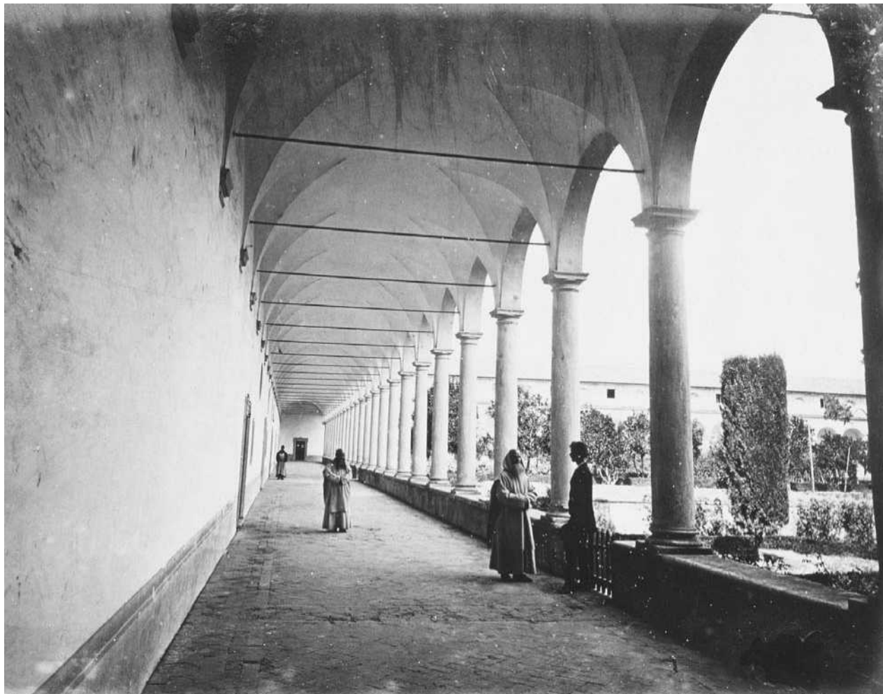
Exterior of portico underside in Cloister of Carthusians, Rome, Italy. (©Michael Maslan Historic Photographs/CORBIS)
