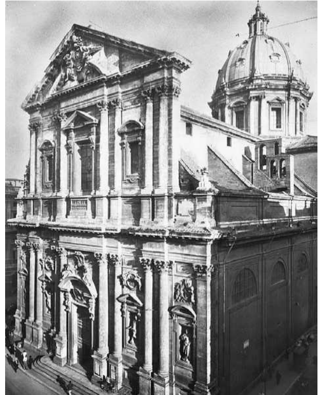
The Church of S. Andrea della Valle, baroque style, with façade designed by Carlo Rainaldi, built 1661–1665, Rome. (Alinari-Art Reference/Art Resource, NY)
